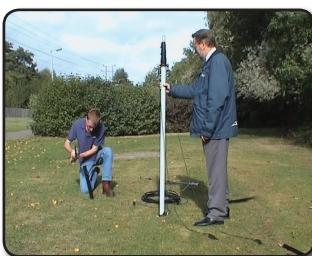
Installing the guy kits using hammer and stakes. (Supplied)
